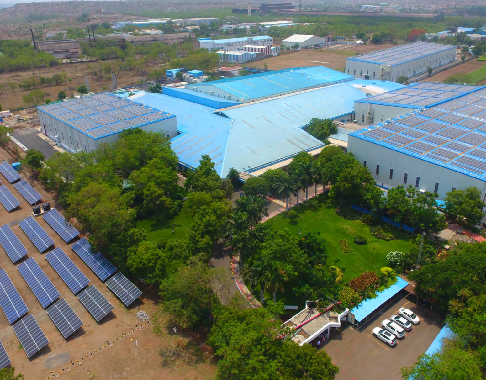
Solar technology installation at our Pune India facility.
